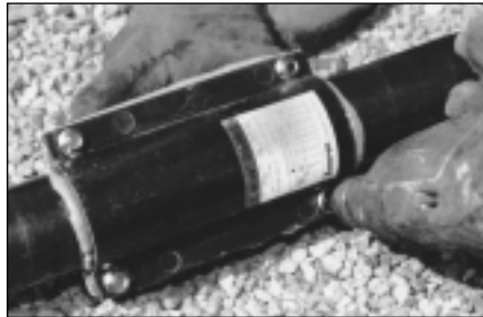
Fig. 8. Join the coupling halves using an Ameron Rivetool. If using bolts, tighten them evenly. A bead of adhesive should be visible between the pipe and the ends of the coupling and between the flanges.
