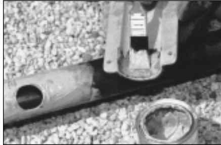
Fig. 6. Apply adhesive to the rim of the hole and to all bonding surfaces.
